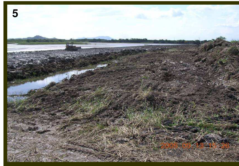
4. Bulldozer removing silt to reinstate areas of open water
