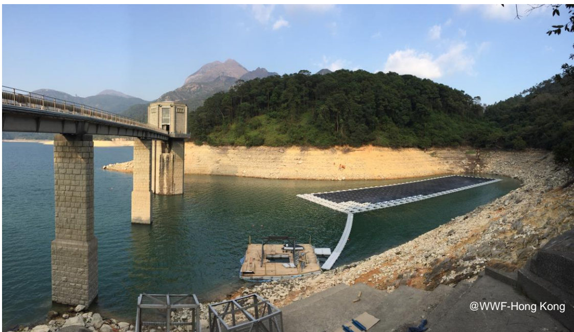
Floating Solar Power System at Shek Pik Reservoir
