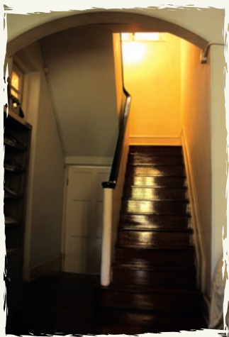
主建築物內的樓梯 Staircase in the main building
